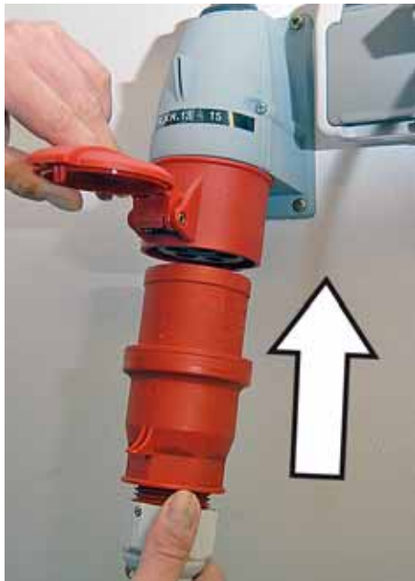
Fig.23: Connecting welder to power supply
